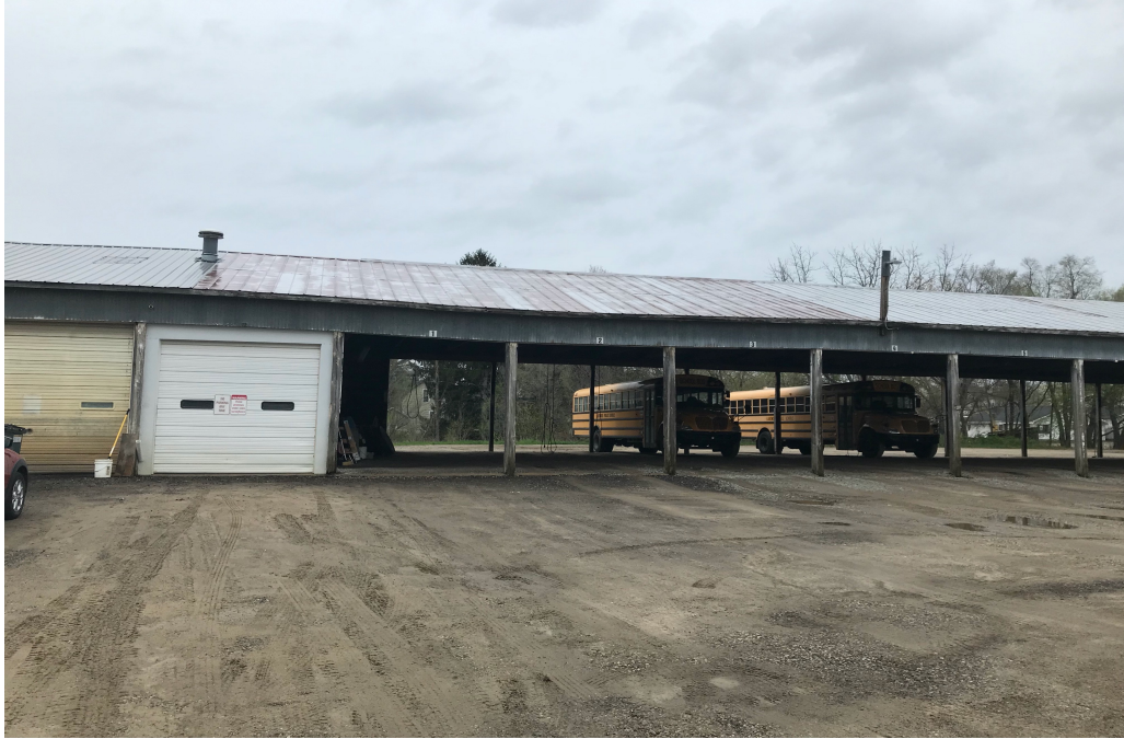
Current bus garage
