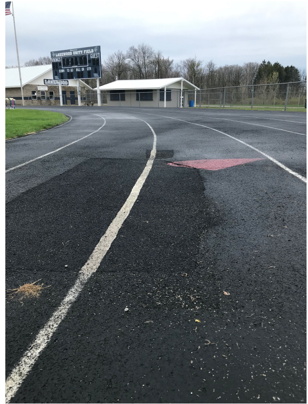
Cracking and sinking at LHS track
